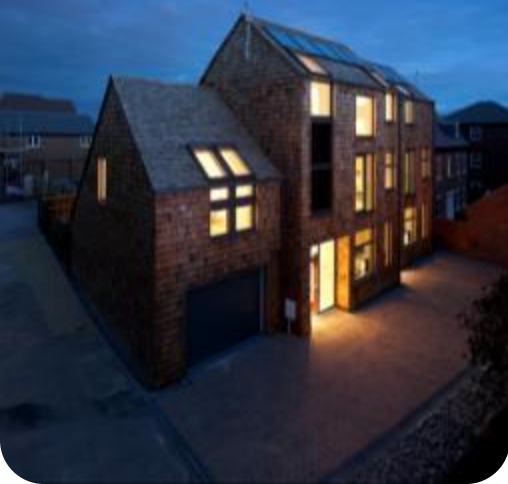
Carbonlight Homes, UK
